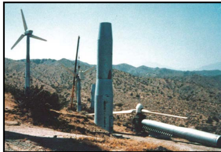
North Palm Spring, CA Earthquake 1986 - damaged wind turbine (EOECAT, 1986)
