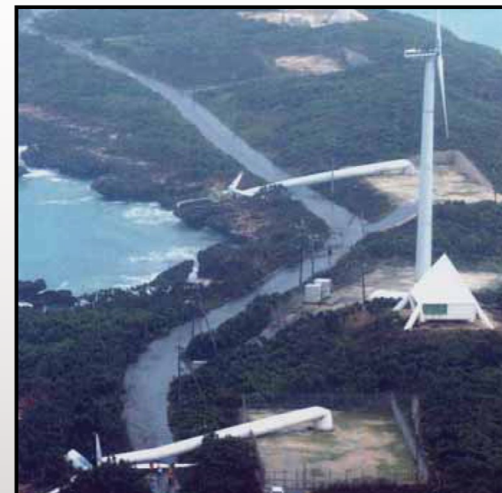
Typhoon Maemi, Japan 2003 - damaged wind turbines (Ishihara et al., 2005)
